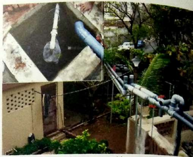
Fig. 5. Roof top harvested rainwater is used for ground water recharge at a residential apartment building in Worli, Mumbai
