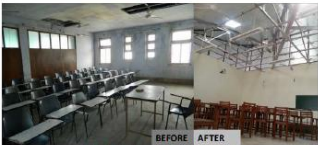
Figure 2: Photo of Classrooms before and after retrofit
