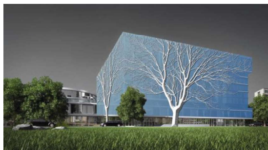
Figure 1: Branching Water Conduits on a Building Facade
